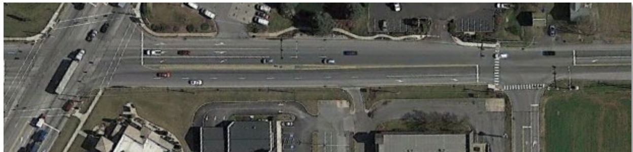
Aerial of PA-896 Improvements at US 30 and Rockvale Road Intersections
