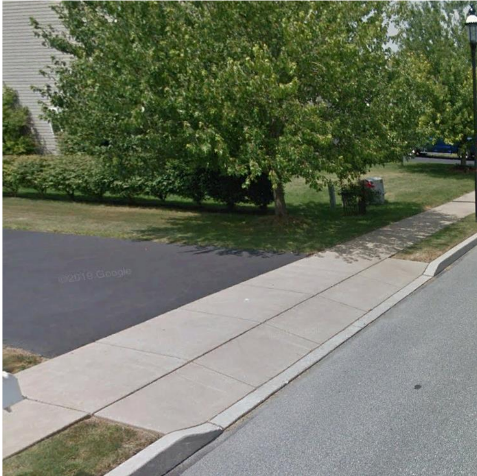
Continuous along the block (recommended for future designs and reconstructions) – Easier for pedestrians, people with mobility or sight issues, or those using wheelchairs or strollers to navigate.
